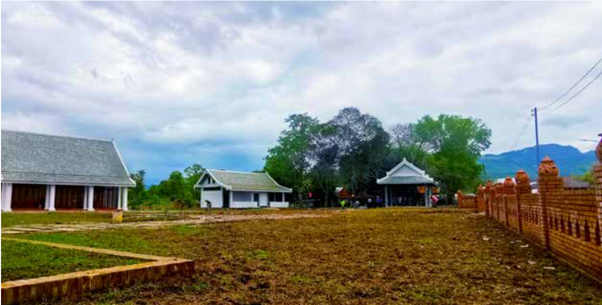
Pottery showcase. The craft display and demonstration center in Ban Chan Neua village, known for its pottery-making for centuries, was constructed and its surroundings landscaped with support from the ADF grant-funded project (photo by Charlene Laxamana).
