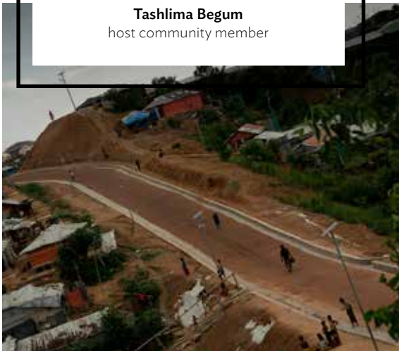
Better access to roads. Displaced persons in the resettlement camps in Kutupalong, Ukhia Subdistrict, Cox’s Bazar District, need roads for safer travels to food distribution centers, health centers, and other facilities (photo by Abir Abdullah).
