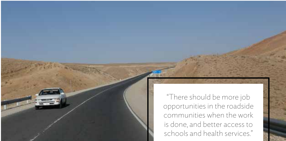
Safer travel. A section of the North–South Corridor Road, rehabilitated with ADF grant assistance, which connects Yakawlang District in the northwest of Bamyan Province to Bamyan City, the provincial seat (photo by Jawad Jalali).
