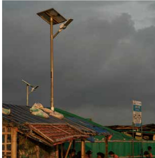
Safer camps. ADB-financed solar-powered streetlights have made the camps safer for residents (photo by Abir Abdullah).
