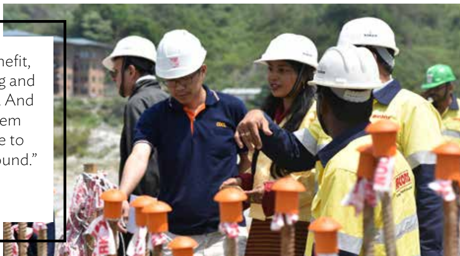
Better urban living. Contractors at the site of the Phuentsholing Township Development Project (photo by Bhutan Resident Mission).
