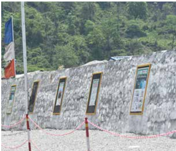
A new township development. Information posters line the walls near the construction site of the Phuentsholing Township Development Project in Bhutan (photo by Bhutan Resident Mission).
