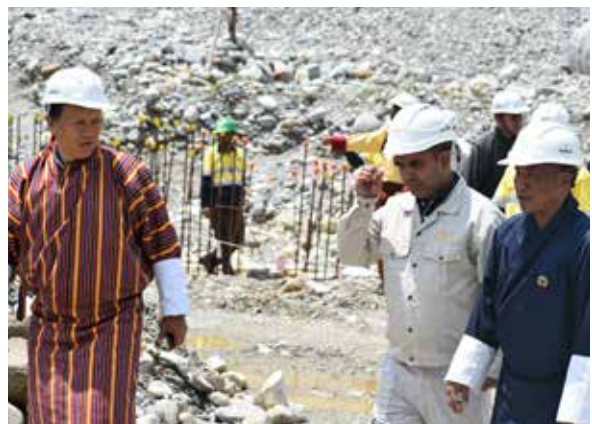
Safeguarding the town. Phuentscholing Mayor Uttar Kamar Rai (right) visits the site of the Phuentscholing Township Development Project where a new urban center will be created (photo by Bhutan Resident Mission).
