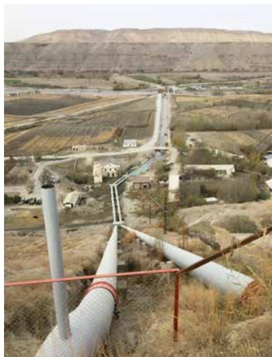
Water pipelines, Aksu Watershed, Tajikistan, ©SDC
