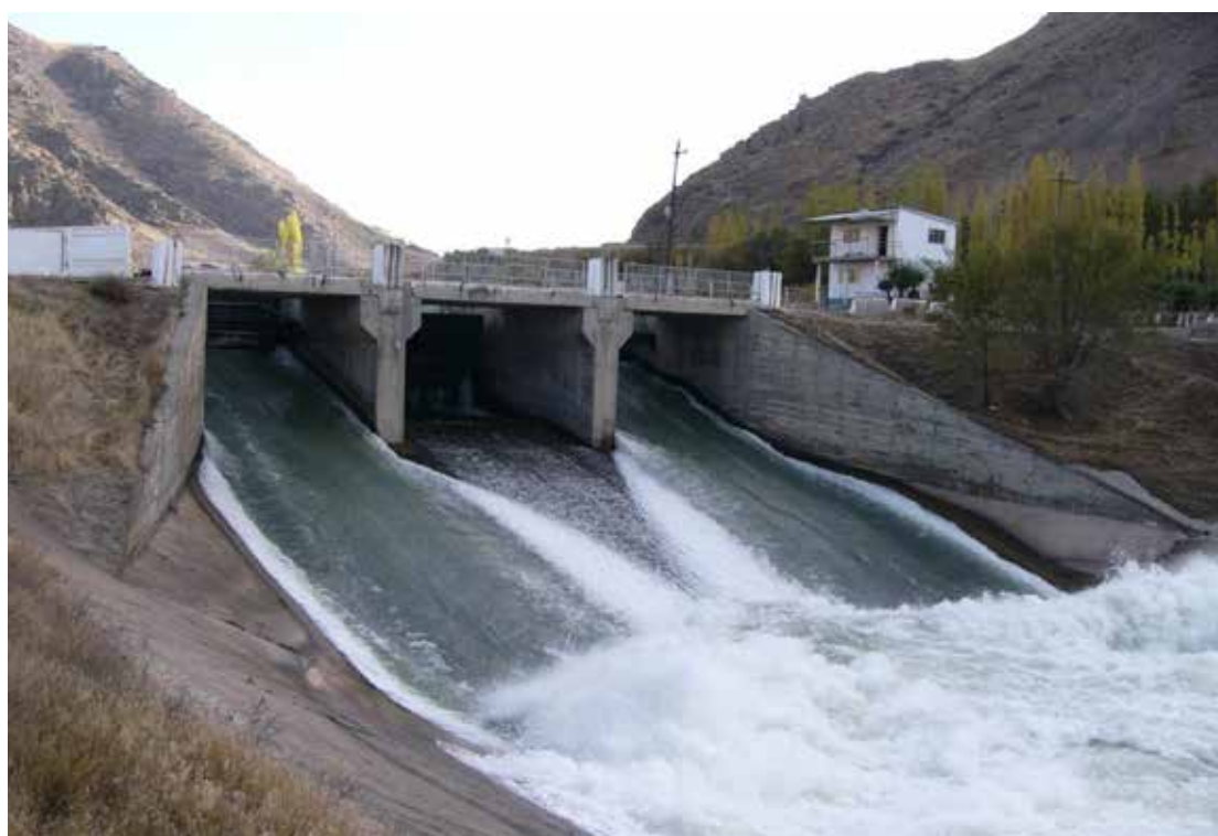
Promotion of Transboundary Water Cooperation between Kyrgyzstan and Kazakhstan: Hydraulic distribution structure below the Kirov reservoir. © SDC
